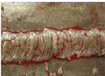
Indication of cracks in a weldment
